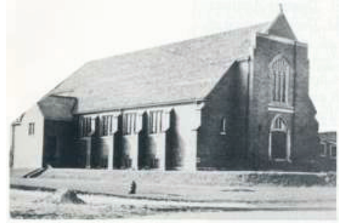
STA PARISH BACK IN 1926!
